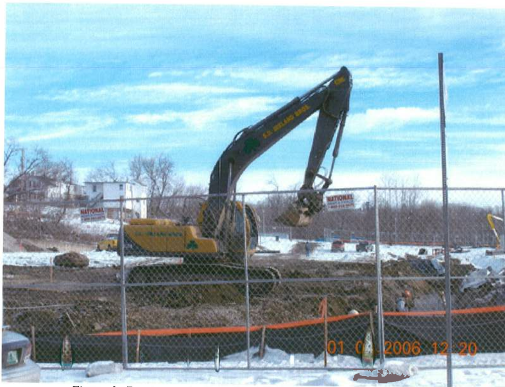
Figure 1: Erosion controls in place at Barlow Place construction site
